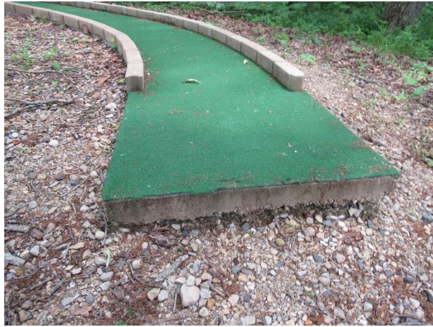
Profile view of concrete slab
