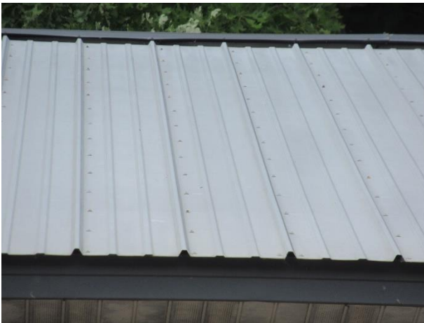
Roof in good condition
