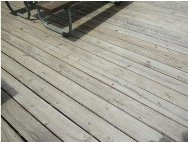
Snack Shack balcony deck boards in good condition
