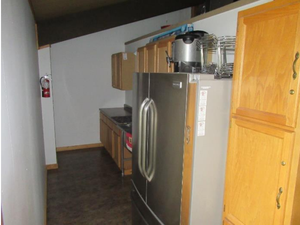
Clubhouse kitchen components
