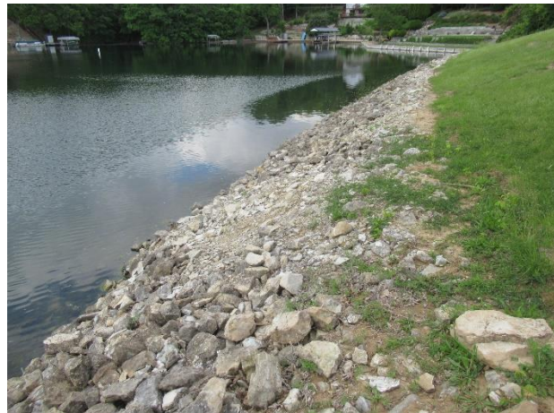
Rip-rap at dam picnic area
