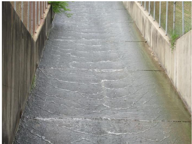
Spillway base concrete in good condition
