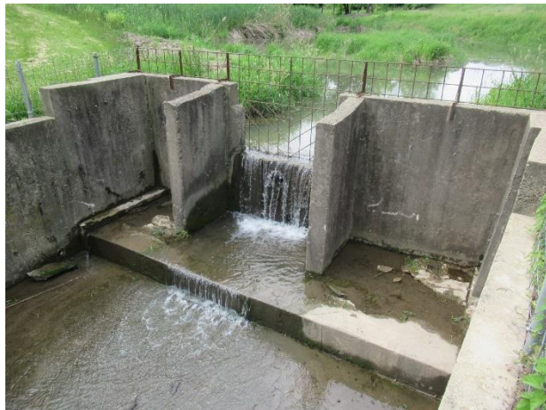
Back side of weir at lake inlet
