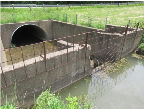
Weir at lake inlet
