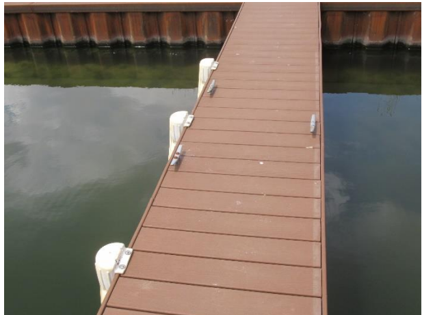
Recently replaced clubhouse dock in good condition
