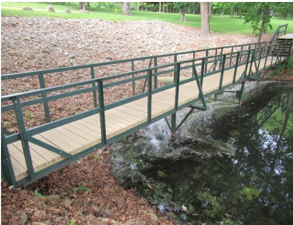
Metal frame bridge at beach dock area
