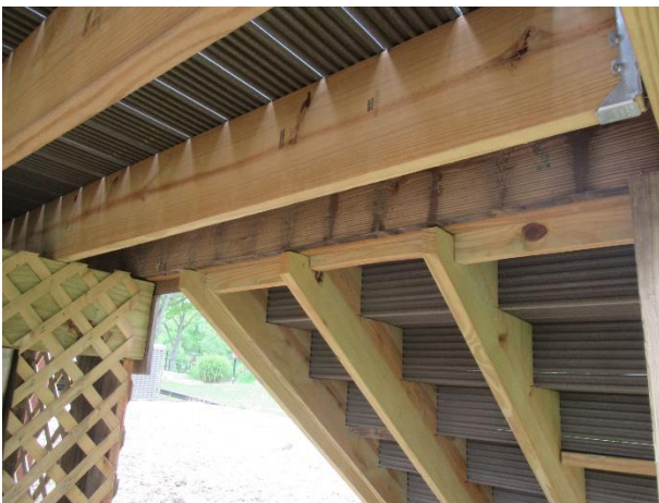
Wood frame structural components at composite balcony and stairs
