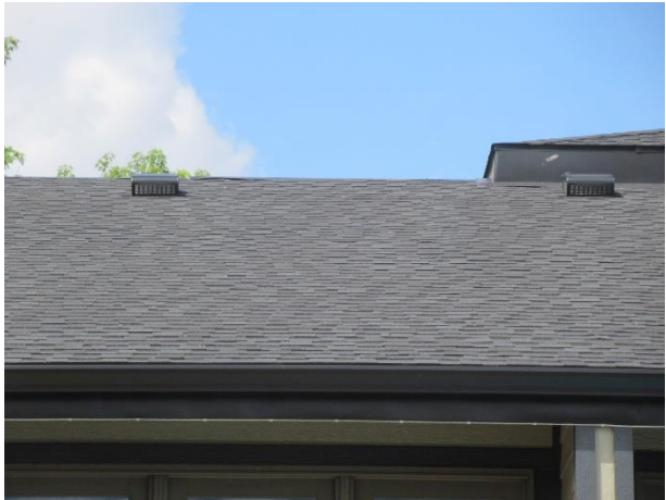
Soffit and box vents at clubhouse roof
