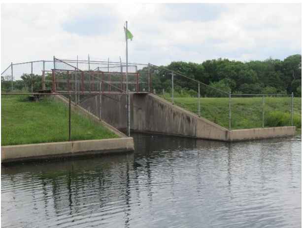
Spillway, fences and bridge
