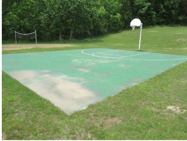
Basketball court overview
