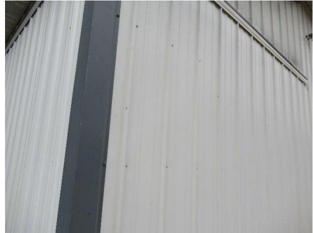
Siding in good condition
