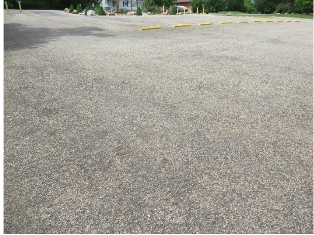
Beach parking area overview
