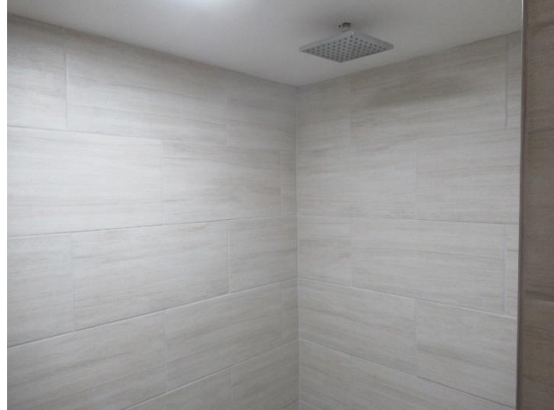
Rest room shower area
