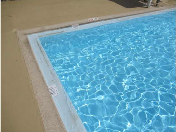
Concrete pool structure with liner
