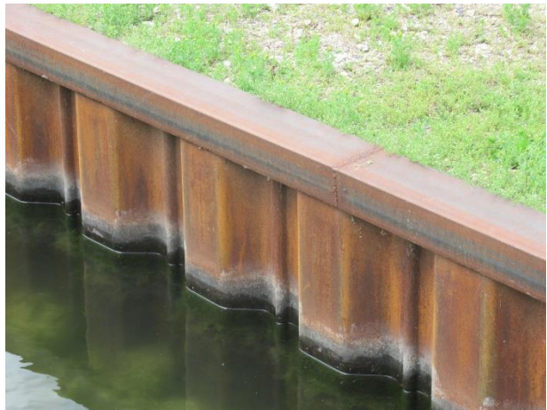
Section of clubhouse dock area bulkhead in good overall condition
