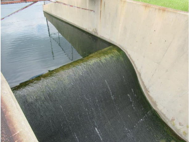
Spillway entrance from lake
