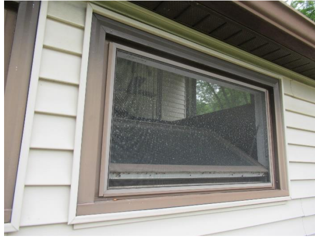
J-channel and operable window at campground shower building
