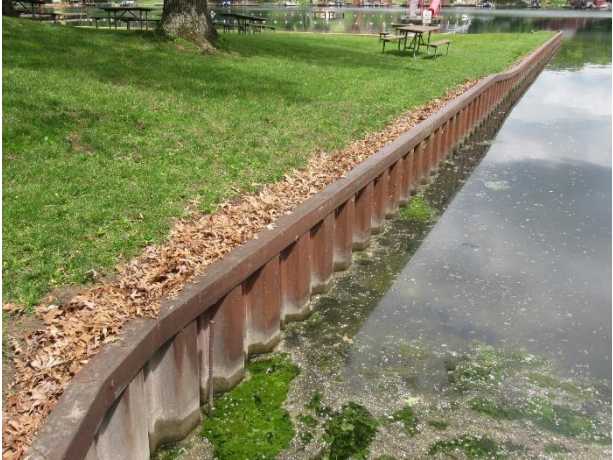
Section of beach bulkhead in good condition
