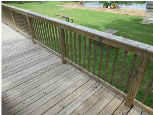
Snack Shack balcony railings in good condition
