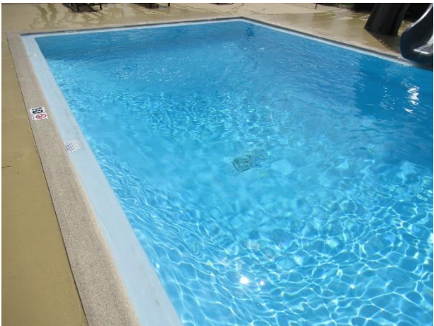
Pool structure with liner
