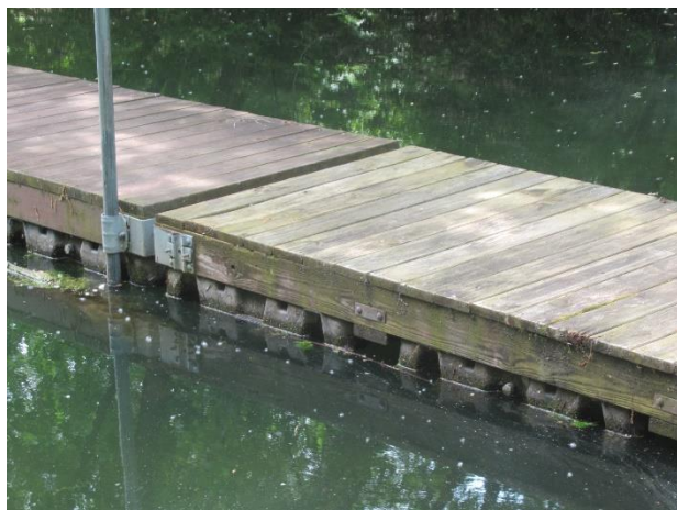
North boat launch floating wood docks with polystyrene billets
