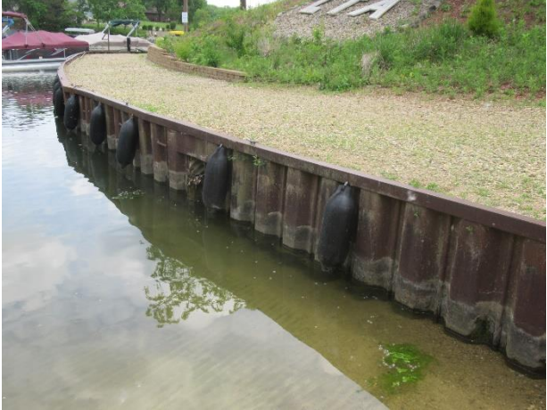
Steel bulkhead at south boat launch
