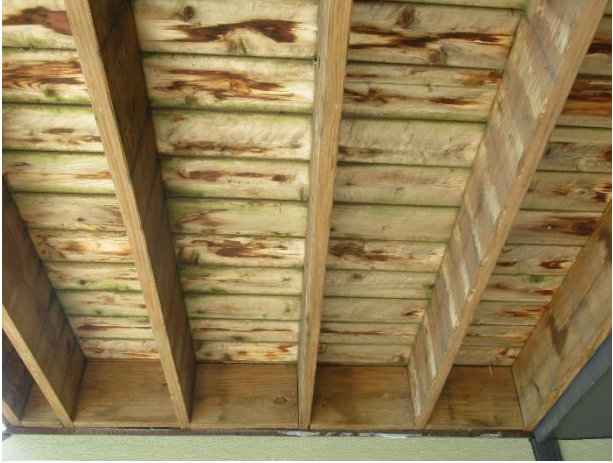
Underside of deck boards and wood joists at clubhouse south balcony in good condition
