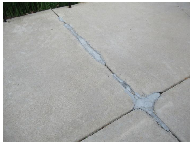
Clubhouse sidewalk repairs
