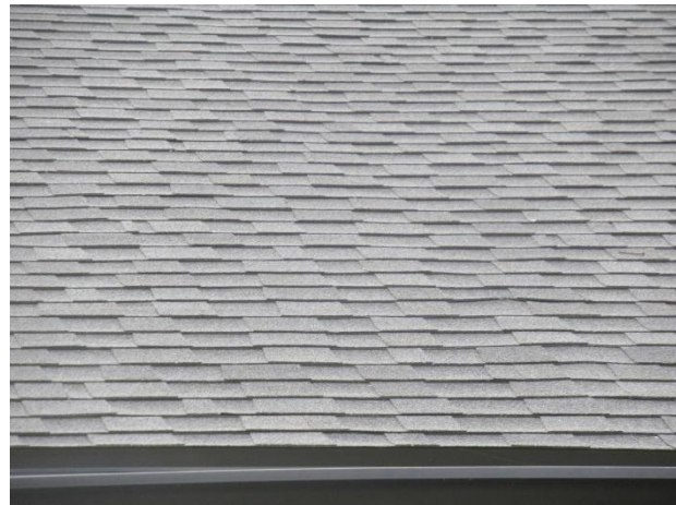
Laminate shingles in good condition at clubhouse roof
