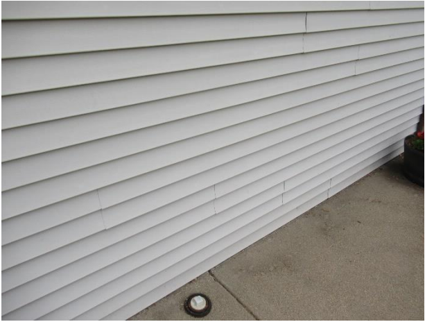
Vinyl siding with a clapboard profile at campground shower building
