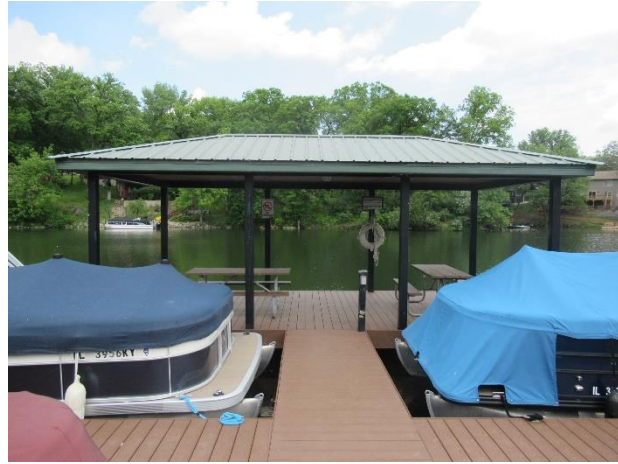
South boat launch dock pavilion
