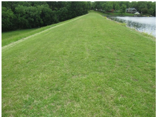
Top side of the dam
