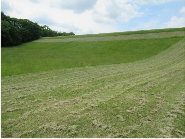
Back side of the dam
