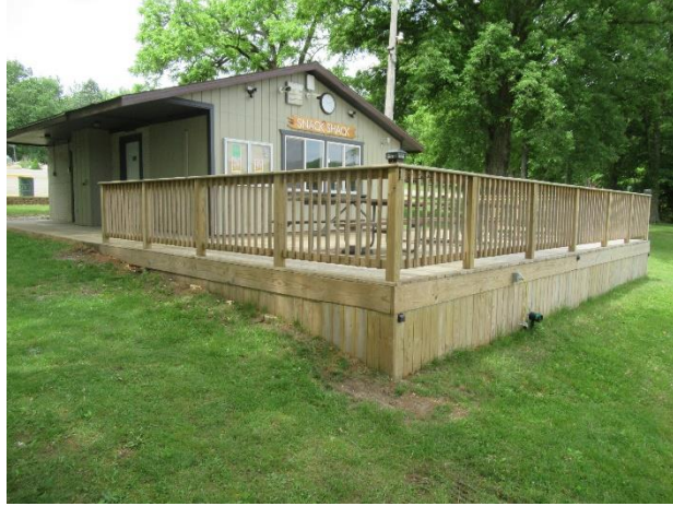
Snack Shack wood frame balcony
