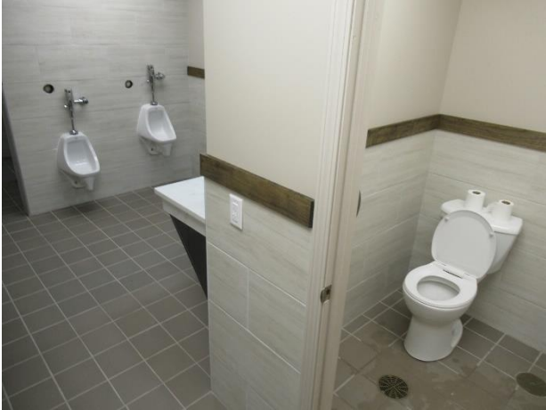
Recently renovated rest room
