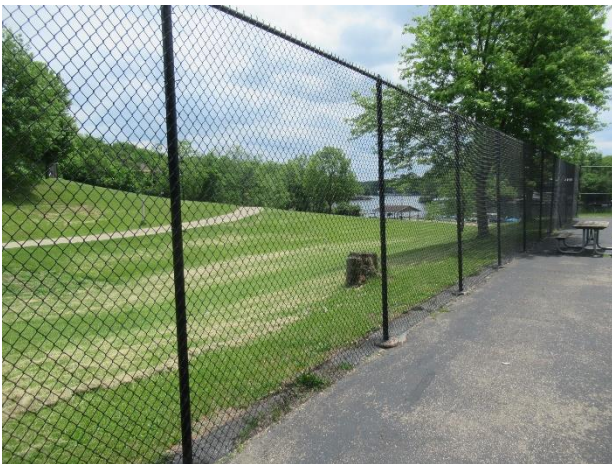
Chain link fence surrounding tennis courts
