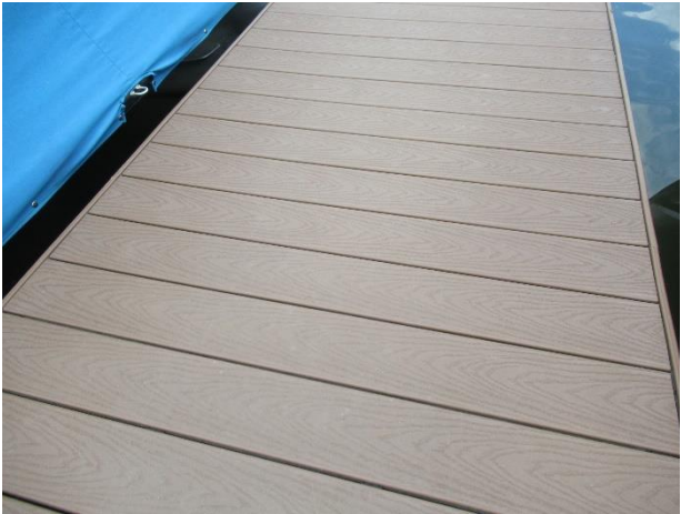
Composite deck boards in good condition
