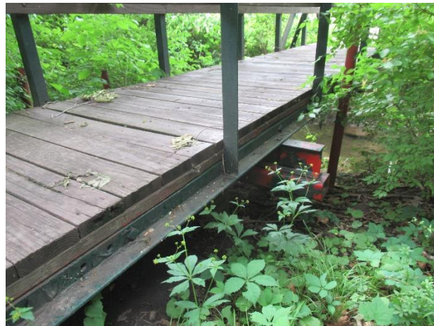
Metal frame bridge at campground
