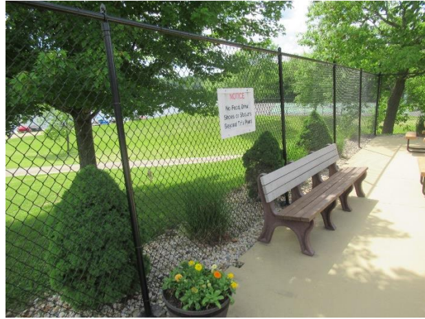
Chain link fencing in good condition
