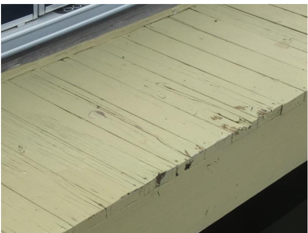
Wood deck board weathering at older section of clubhouse docks
