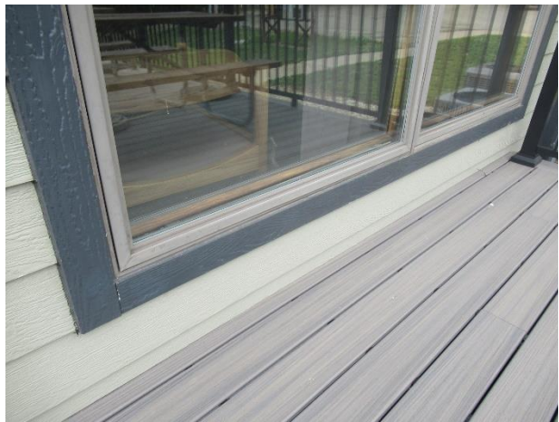
Aluminum frame in good condition
