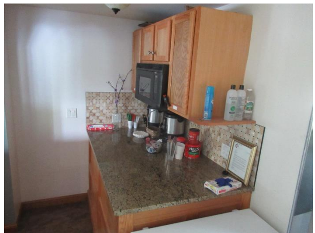
Clubhouse kitchen components
