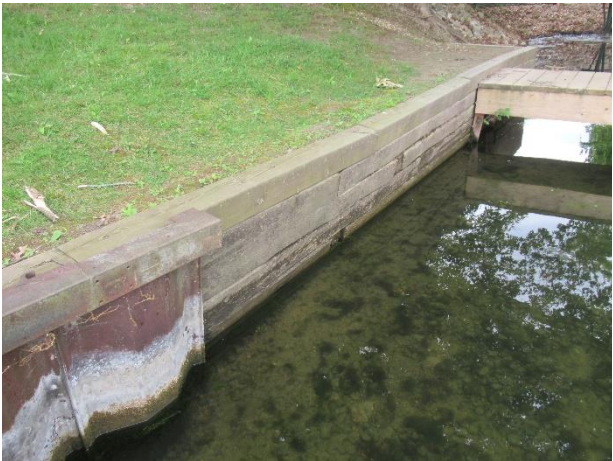
Section of beach bulkhead comprised of wood timbers
