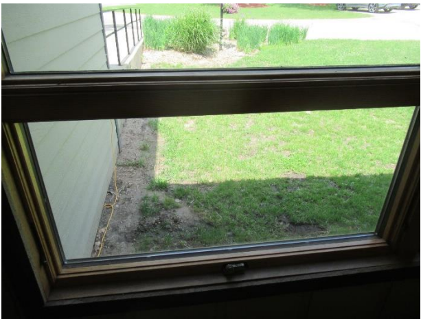
Operable window at upper level
