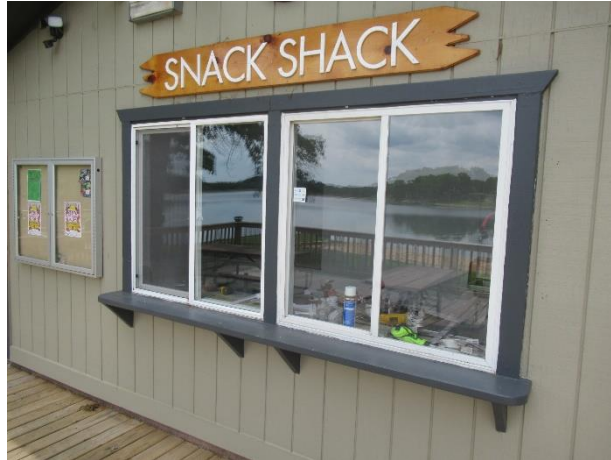
Plywood siding and windows
