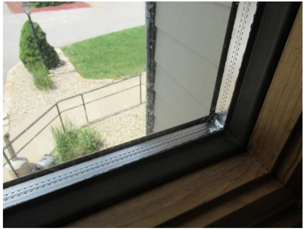
Clubhouse windows with dual pane glass
