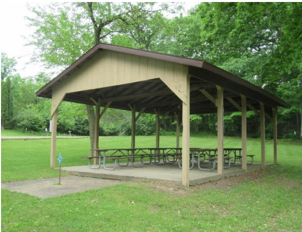
Beach amenity area upper pavilion
