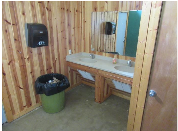
Shower room sinks
