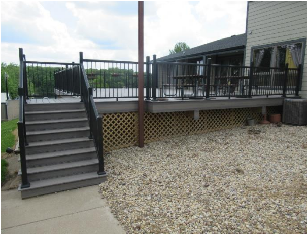
Composite balcony at clubhouse
