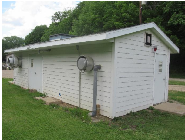
Pump house overview
