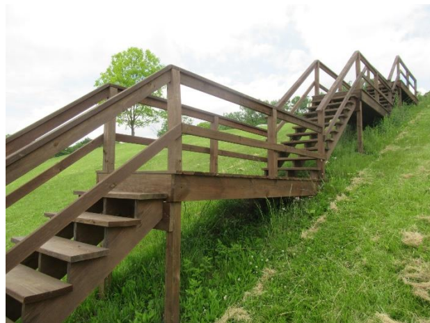
Wood frame stairs between picnic area and dam
