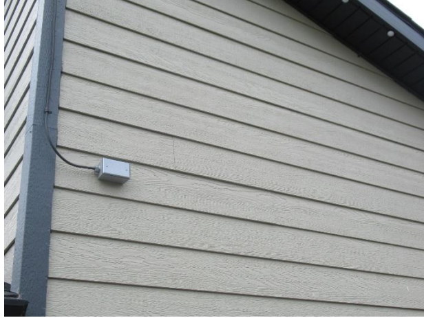
Siding and finish in good condition
