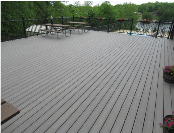
Deck boards in good condition
