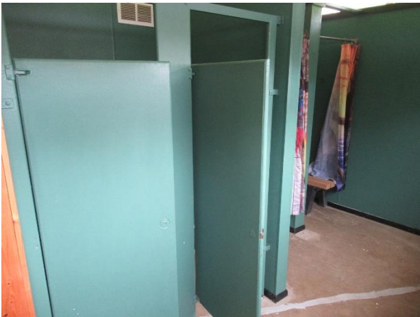
Shower room partitions
