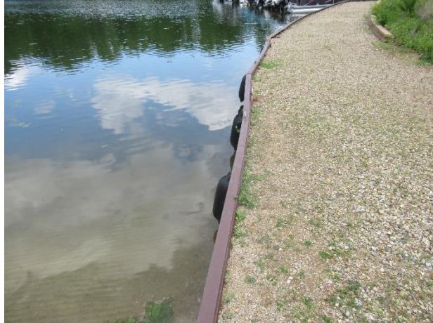
Topside view of south boat launch bulkhead
