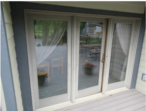
Door and adjacent windows
