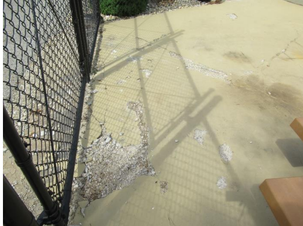
Coating deterioration
