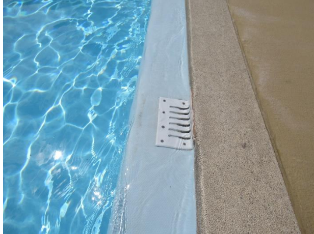
Liner and drain at coping area
