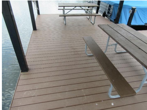
Composite deck boards in good condition
