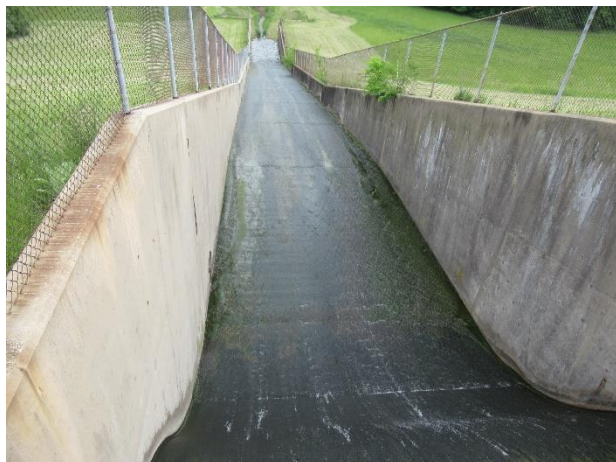
Concrete spillway structure
