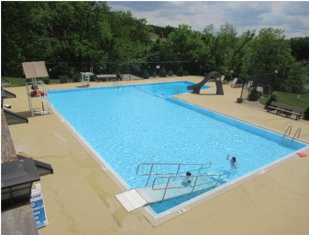
Pool and deck overview
