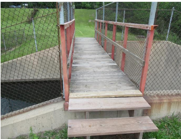
Dam bridge over the spillway
