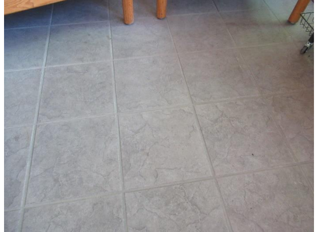
Ceramic tile floor coverings at entry foyer
